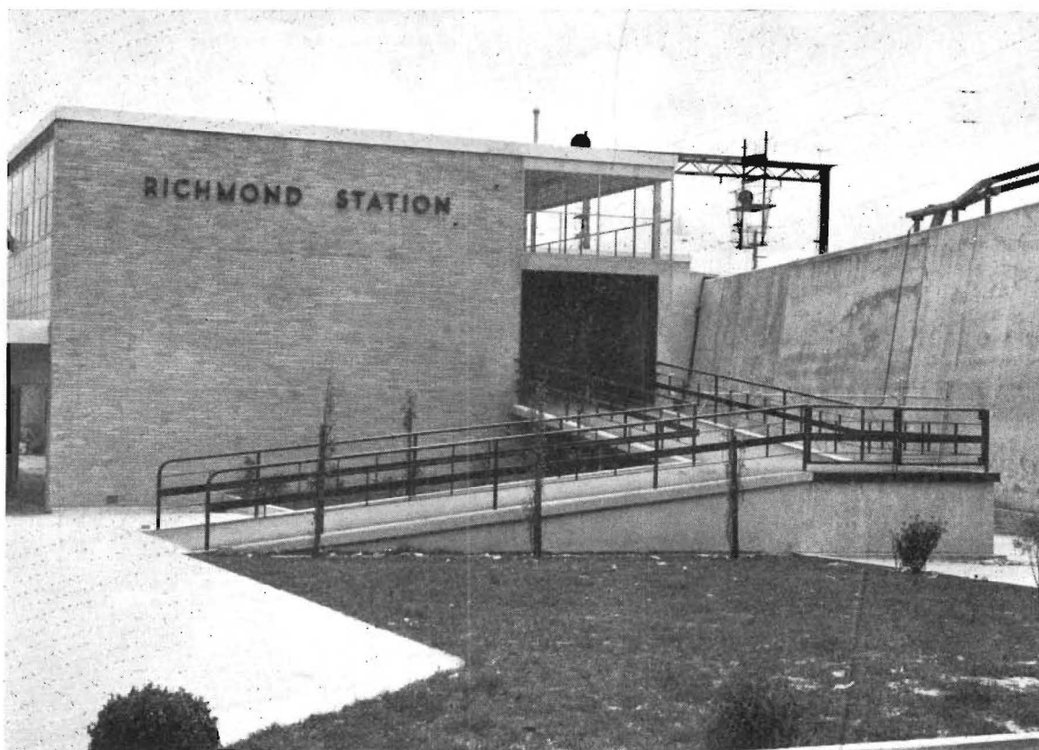
New Richmond station building on Swan Street frontage.
