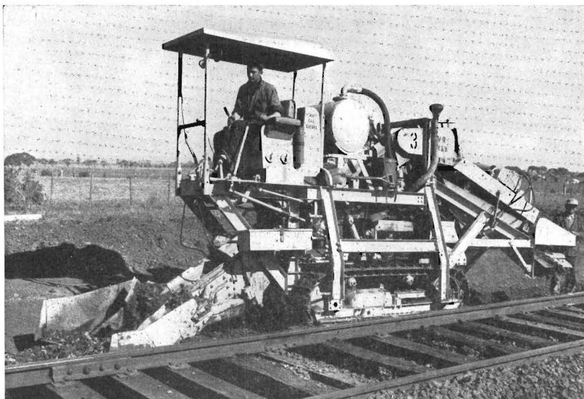
"Super Mole" ballast cleaning machine.
