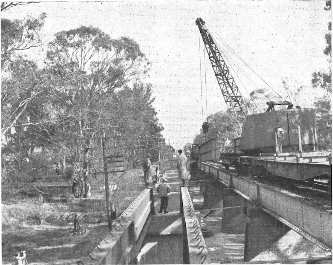
Duplication of bridge for standard gauge line at Seven Creeks, Euroa.
