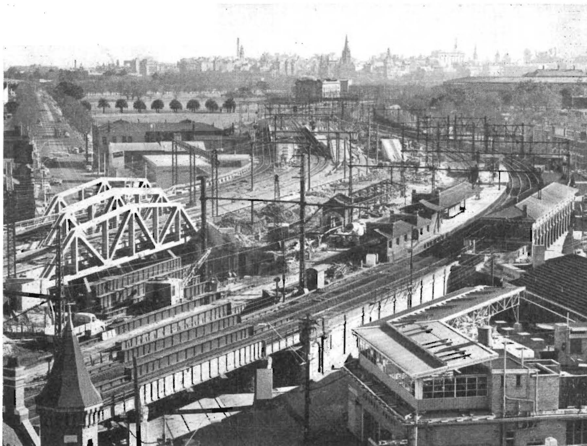
General view of reconstruction work at Richmond station.
